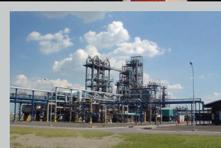
The polypropylene plant at the Safripol complex in Sasolburg. PP production commenced at Safripol in 1974, but here we see the new plant, commissioned in 1997. Spheripol technology from Basell is used.
